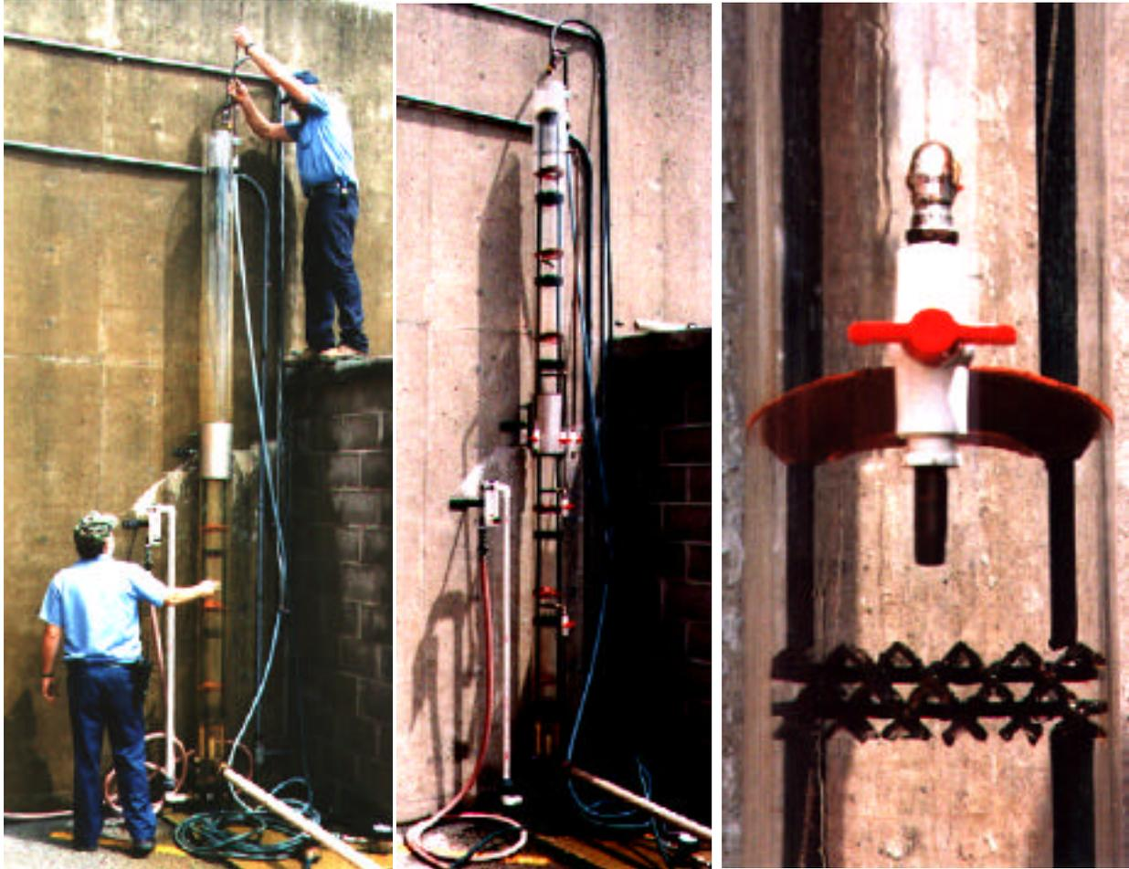
**Construction of Tower Aerator and Installation of Iron Gratings Designed and Fabricated at Normal**
