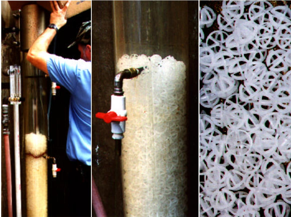
**Installation of Plastic Packing in Tower Aerator**
