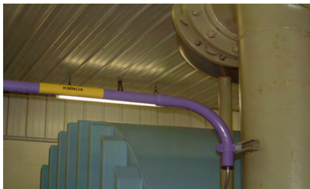
Permanganate is added to aerated water (filter influent) to oxidize manganous ion ( Mn^{++} ) to Mn(OH)_4 , a brown-black precipitate.
